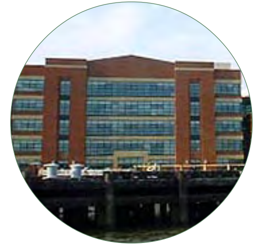
Naval District Washington, located at the historic Washington Navy Yard next to the Anacostia River in the District of Columbia, adopted Low Impact Development (LID) to decrease its impact on the Anacostia river. Photo: CONCERN, Inc.
